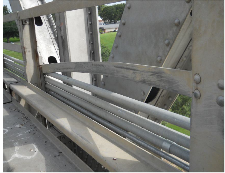
Middle rail at panel point L80, upstream
