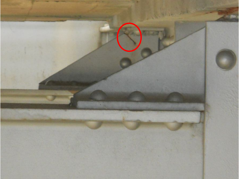
Knee brace at Stringer 3, panel point L32
