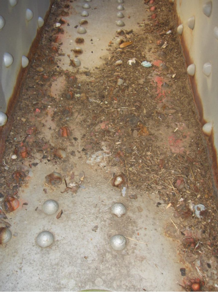
Typical defective rivets, inside box of the lower chord
