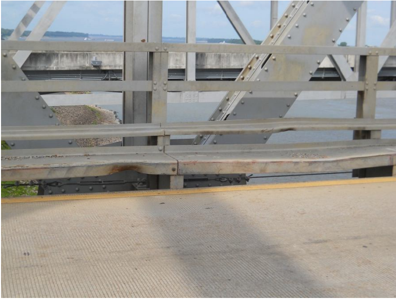
Upper and lower curbs at panel point L6, downstream
