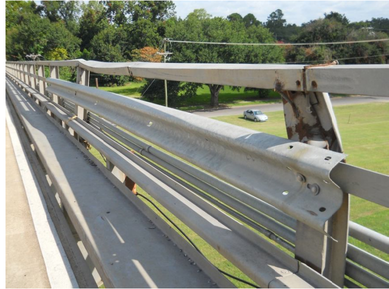
Top rail, middle rail and posts at west approach, downstream
