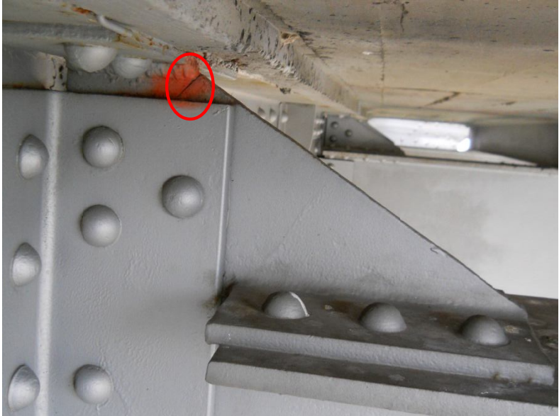
Knee brace at Stringer 3, panel point L52
