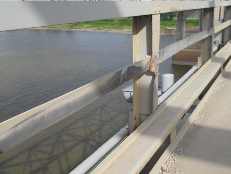
Post between panel points L40 and L41, downstream
