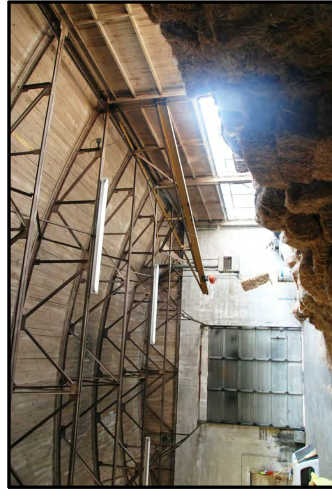
PHOTO - 3A ITEMS IN THIS PHOTO WILL BE DEMOLISHED BY OWNER UNDER SEPARATE CONTRACT PRIOR TO CONSTRUCTION.
