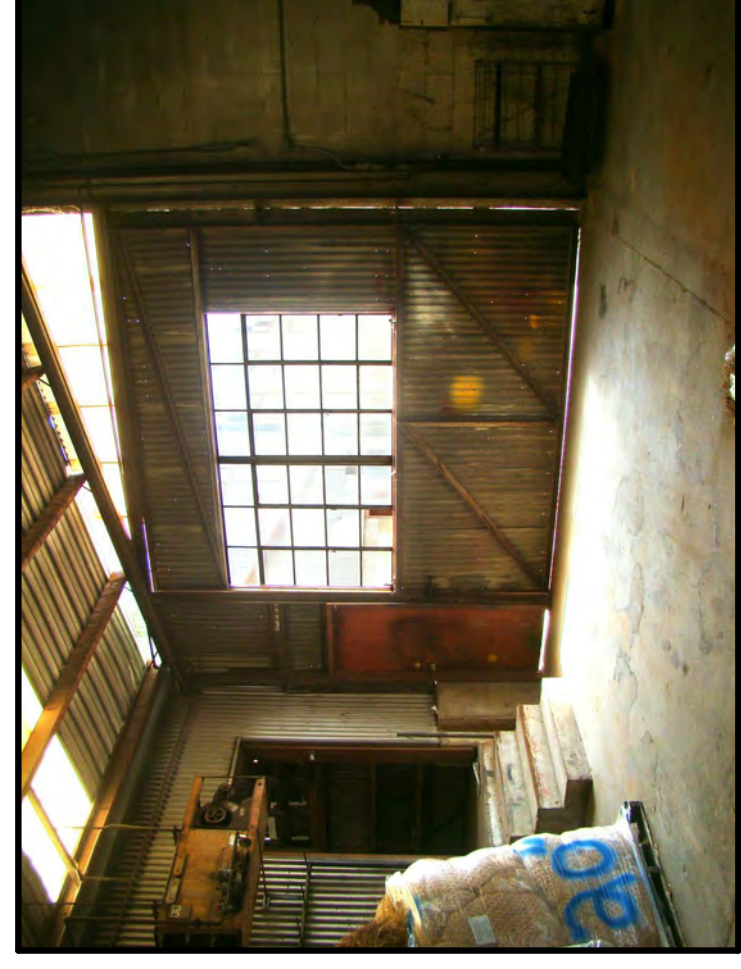
PHOTO - 3F MOST ITEMS IN THIS PHOTO WILL BE DEMOLISHED BY OWNER UNDER SEPARATE CONTRACT PRIOR TO CONSTRUCTION.
