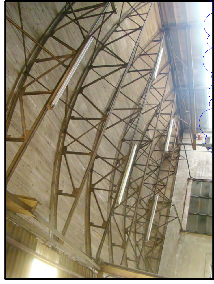
PHOTO - 3D ITEMS IN THIS PHOTO WILL BE DEMOLISHED BY OWNER UNDER SEPARATE CONTRACT PRIOR TO CONSTRUCTION.
