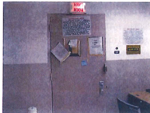
Material 030, Fire Door Lining, Inaccessible Core, 1-1/2" Thick, Tan, Painted, Metal First Vault Door
