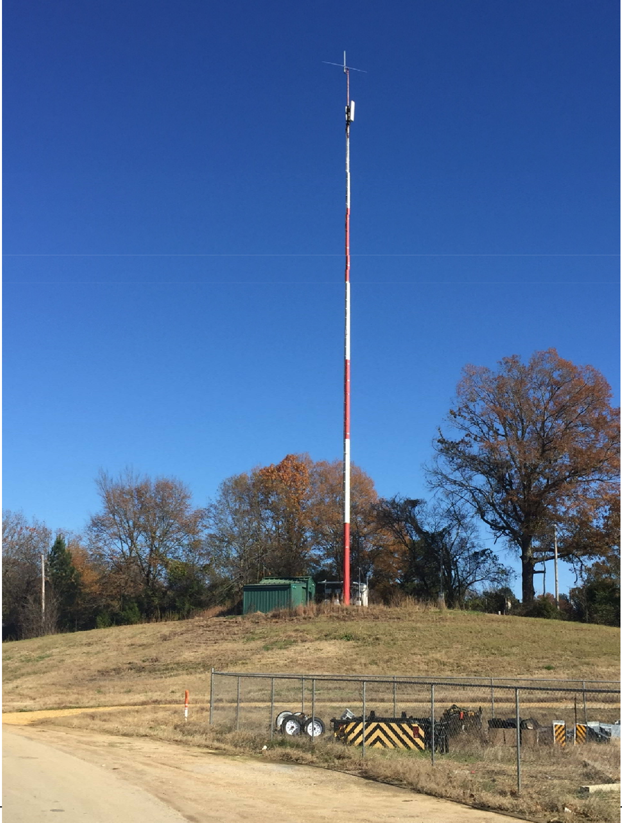
PHOTO OF EXISTING MAIN TOWER SITE:
