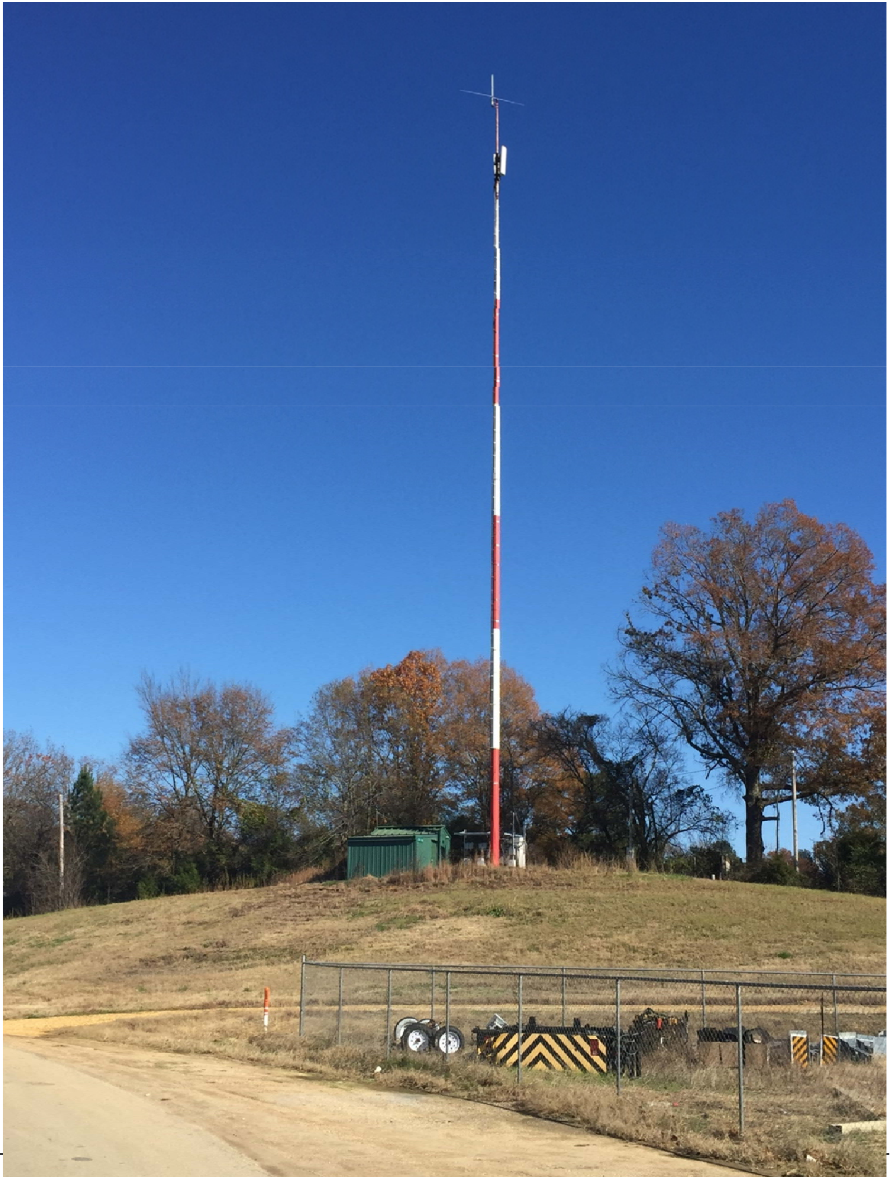
PHOTO OF EXISTING MAIN TOWER SITE:
