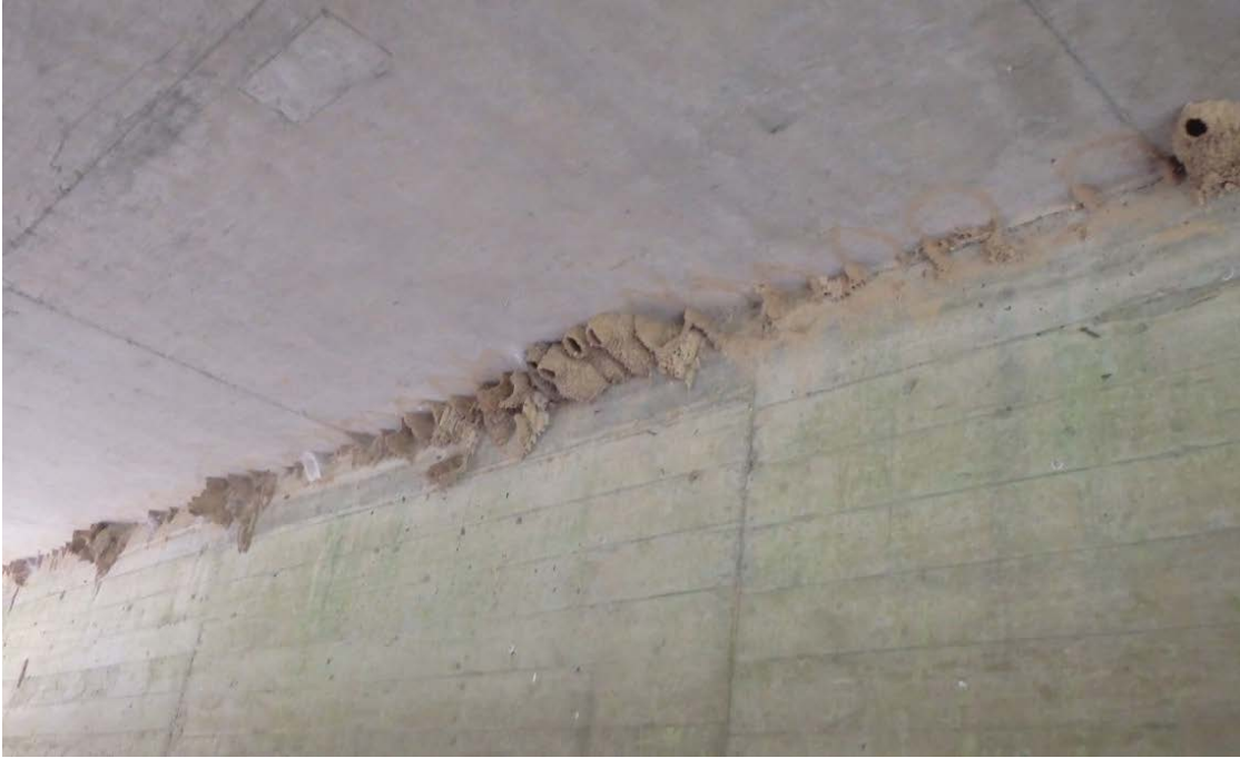
Cliff swallow and barn swallow nests in a culvert. Photo: USFWS
