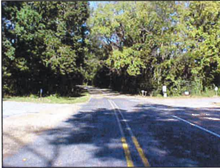
Willows (Willow Springs). Old Port Gibson Road in center, Willows Road to left, historic Natchez Trace to right.
