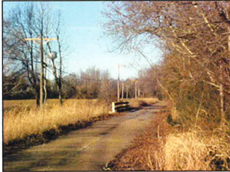
Old Fourteenmile Creek Bridge, Raymond Military Park
