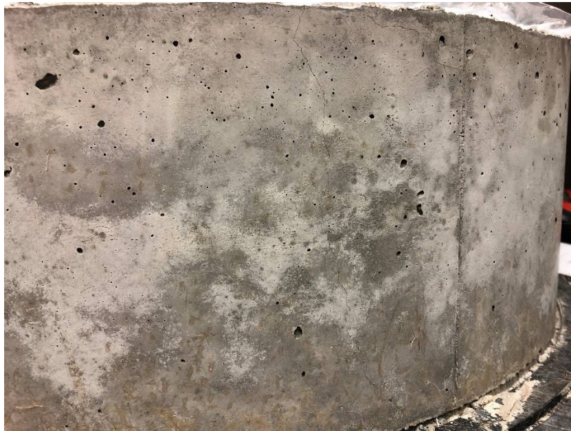
Figure 14. Drying Shrinkage Crack – Mix 3, Ring B
