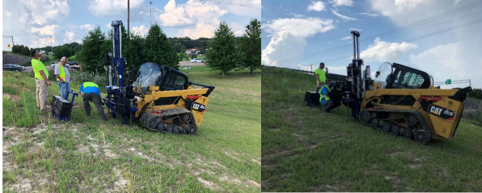
Figure 3.11 Field Activity of CPT test at Slope 2
