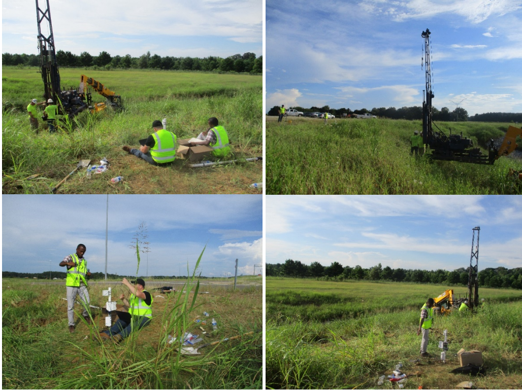
Figure 4.48 Installation of sensors at Slope 5
