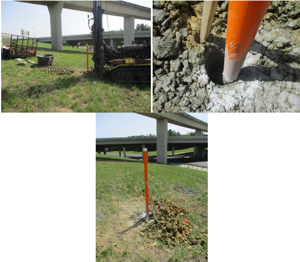
Figure 4.6 Slope 1 slope inclinometer installation
