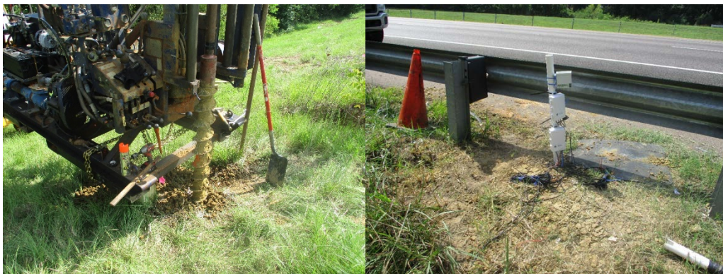
Figure 4.38 Field installation of the sensors at Slope 4
