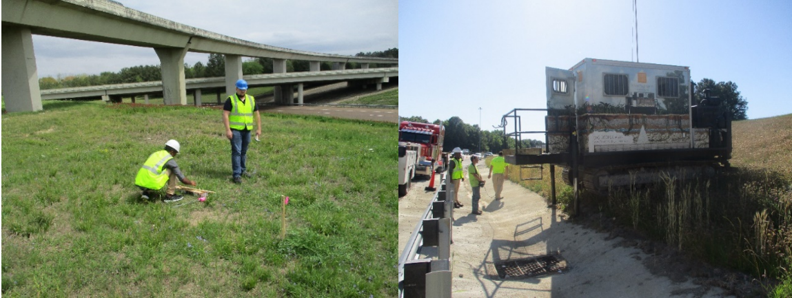
Figure 3.3 Conducting CPT test at Slope 1
