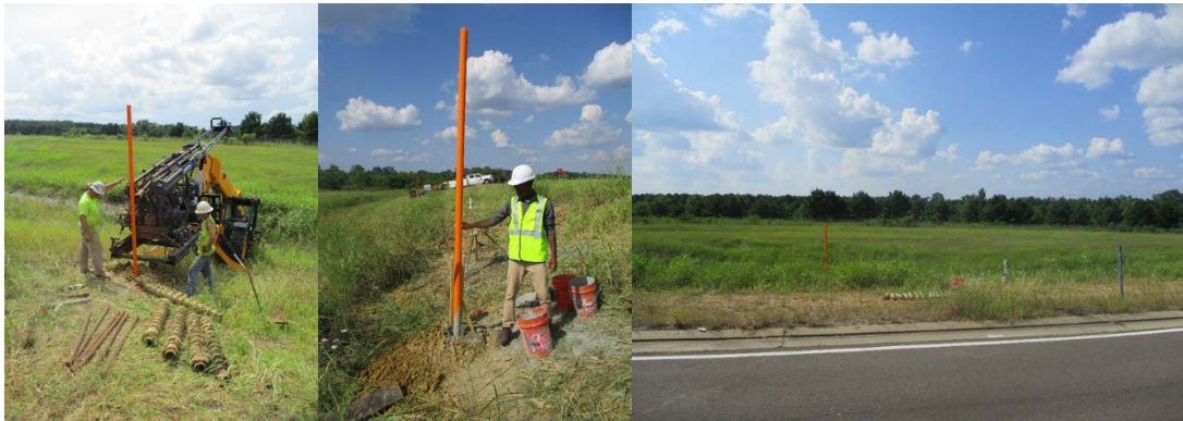
Figure 4.49 Slope 5 slope inclinometer installation
