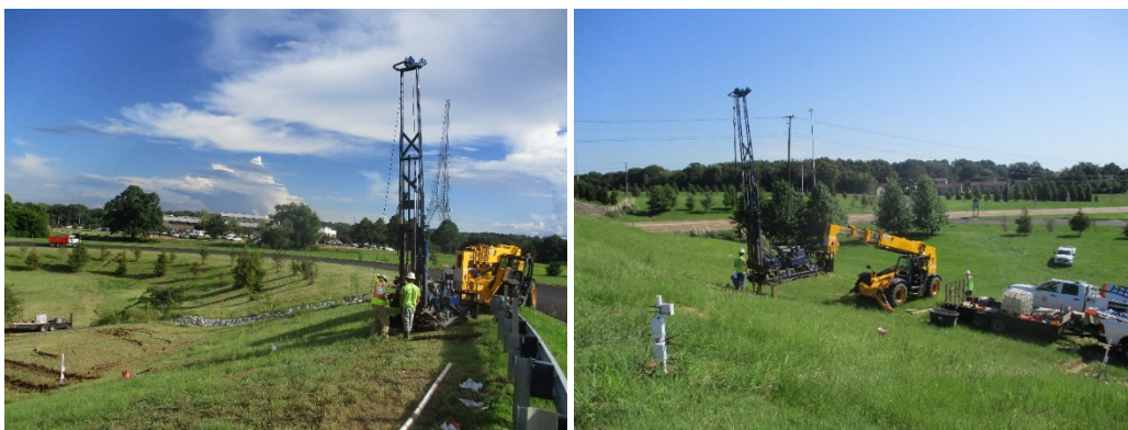
Figure 4.16 Field Activities photo at Slope 2.
