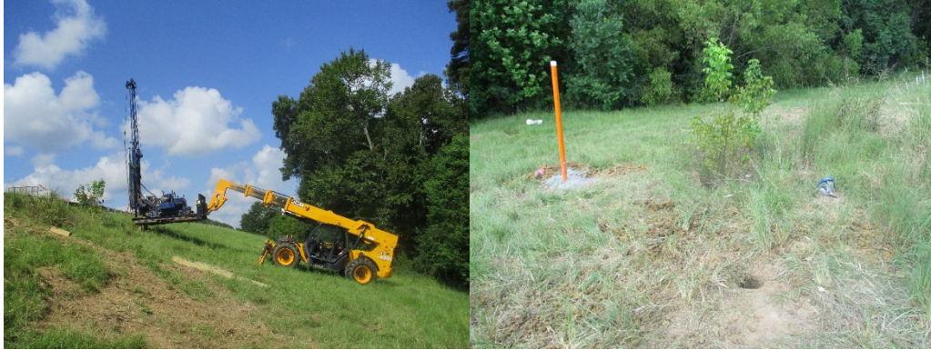
Figure 4.39 Installation of vertical inclinometer at Slope 4
