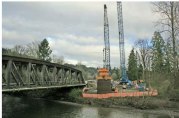
Contractor crews working for WSDOT in the process of rebuilding a new bridge on State Route 162 across the Puyallup River Bridge in Pierce County.
